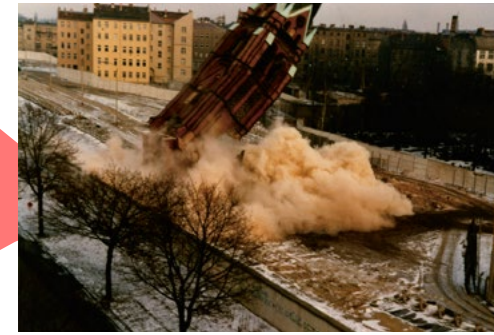
Demolition of the Reconciliation Church, Bernauer Strasse, 1985 Photo: Krüger
